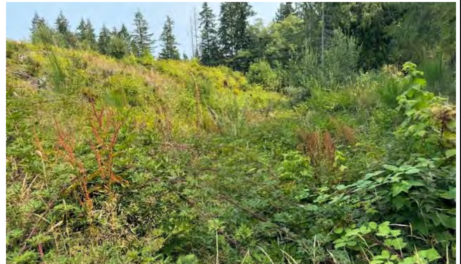
Photo 32 -lower ditch along north segment road.
