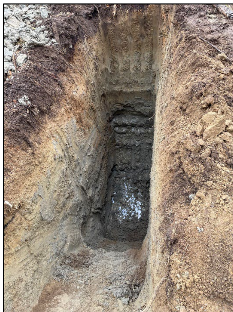
Photograph 1: Exploration pit EP-15 with groundwater seeps between depths of 8.0 to 9.0 and 10.5 to 11.5 feet bgs.
