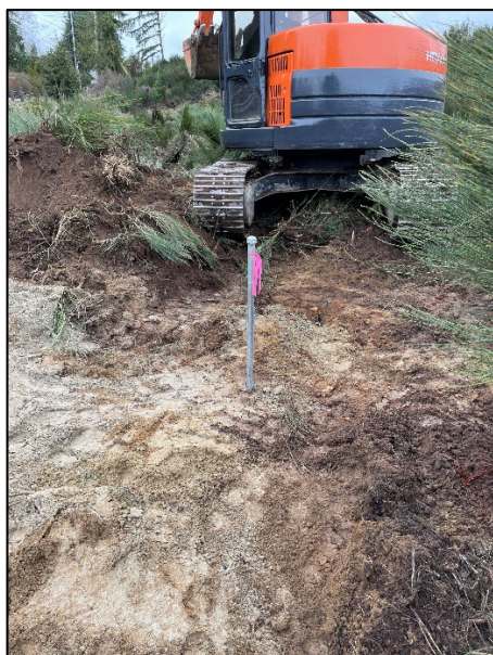
Photograph 2: Well point WP-2 located approximately 15 feet northwest of exploration pit EP-18.
