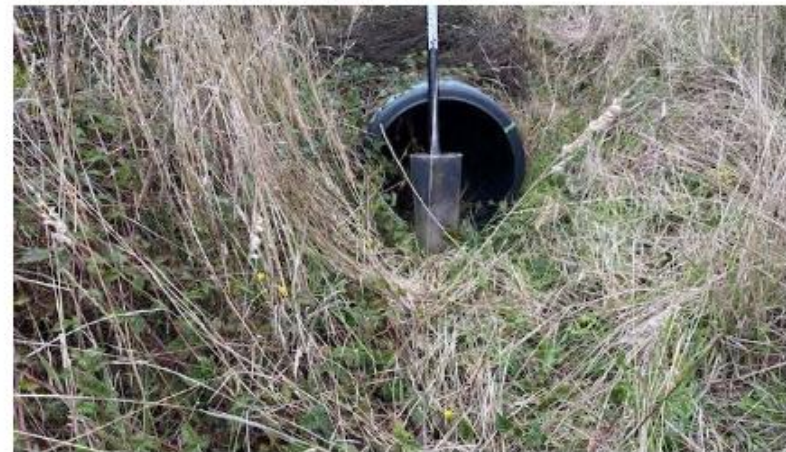
Photo 36 shows a culvert under one of the service road. It appears that the culvert was installed during construction of logging roads.
