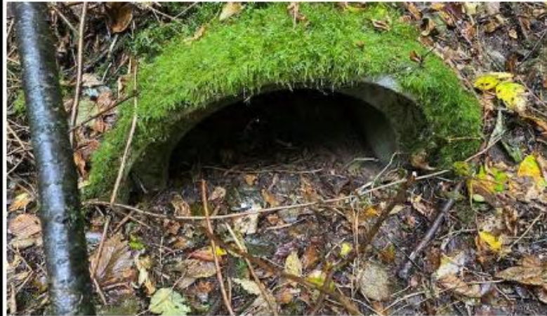
Photo 35 shows the culvert under Bond Road at the north end of the South Segment.
