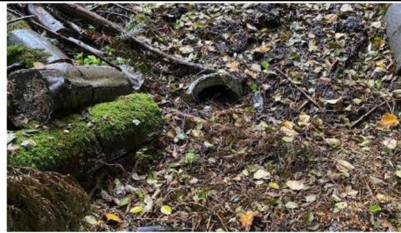
Photo 34 shows the culvert under Bond Road in the upland between Bond and Stottlemeyer Roads in the south segment.
