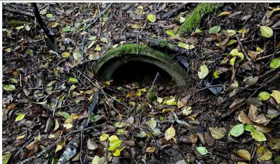
Photo 33 -Shows the inlet of the culvert under Stottlemeyer Road, which is at the end of the non mapped stream just west of the road.
