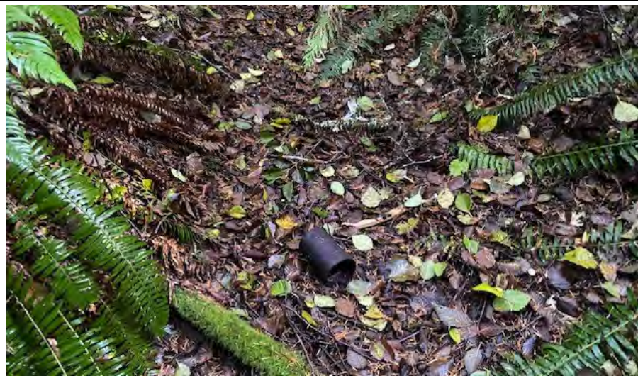
Photo 10 -Test Plot 20 looking north toward culvert under Stottlemeyer Road. Bare ground with no evidence of water flow.
